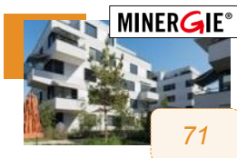
Regensdorf (Sonnenhof) Schulstrasse 95/97/99/101/103/105
